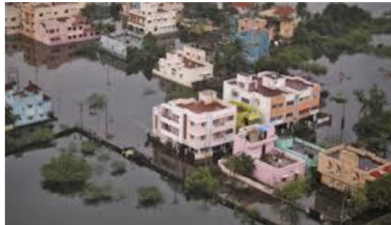
Flooding in Chennai [Source: Oxford Analytica]
